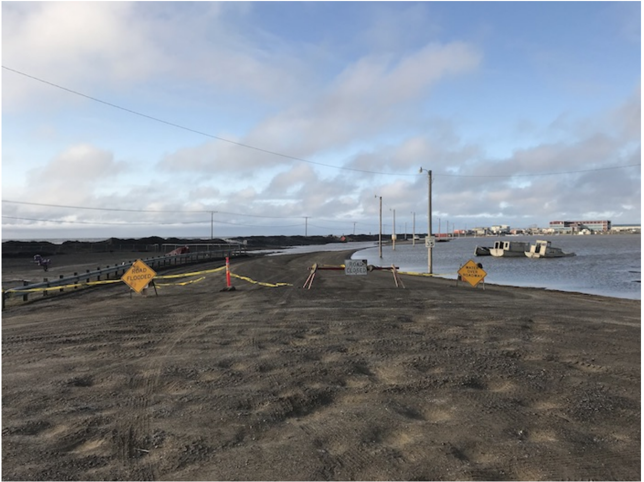
Figure 5. Photo from Utqiagvik, Alaska in early August 2019 during a strong westerly storm that caused flooding and closure of Eben Hopson Street one of the primary roads in the community. Photo courtesy of Benjamin Jones.
