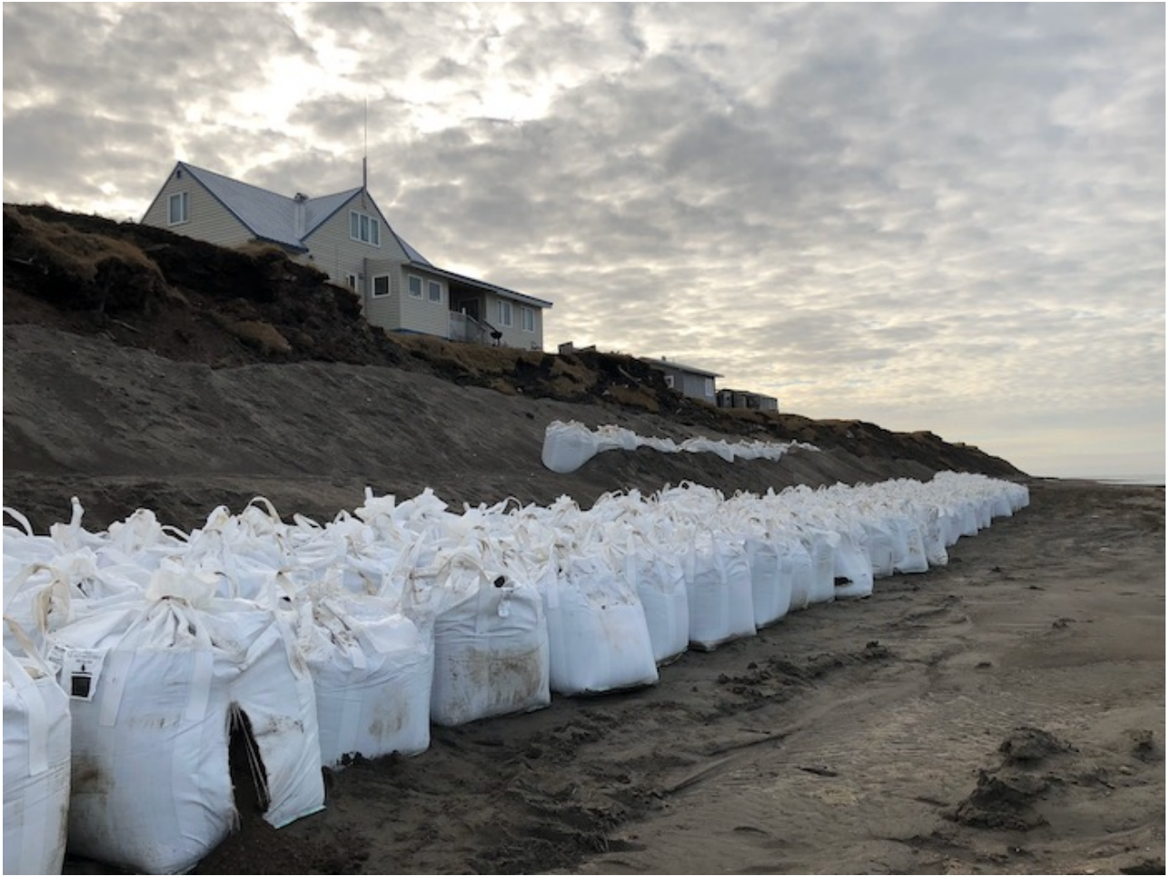
Figure 4. Photo from Utqiagvik showing erosion mitigation measures being utilized to mitigate impacts of erosion to permafrost coastal bluffs and houses that sit atop the bluffs. Photo courtesy of Anne Jensen.
